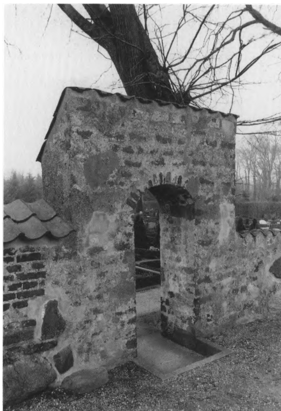
Fig. 3. Portal i kirkegårdsmuren nord for kirken (s. 2121). NE fot. 1990. - Gate in the northern wall of the churchyard, seen from the outside.
